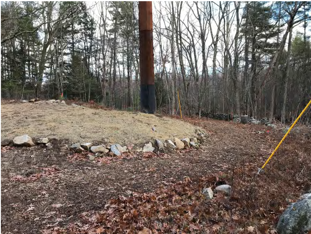
Fig 8: Str. 90 work area. Viewing north. (11-16-20)
