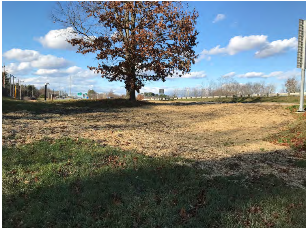
Fig 10: Graded and straw mulched access to Strs. 130 and 129 work area. Viewing north. (11-17-20)
