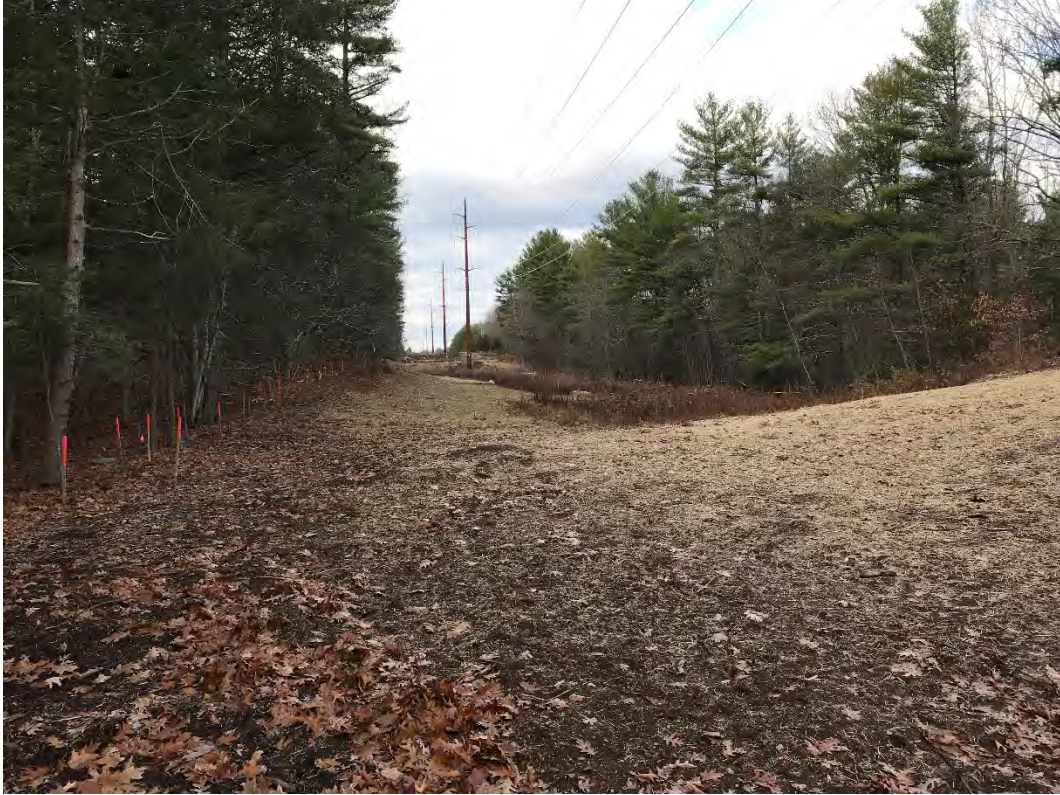
Fig 9: Graded and straw mulched access route between Strs. 90 and 89. Viewing northwest. (11-16-20)
